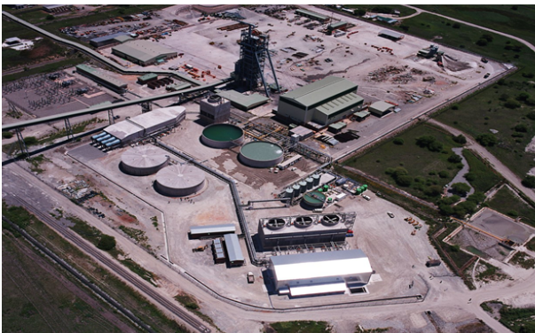
Amandelbult Ammonia Refrigeration Plant - 21mW(R)
